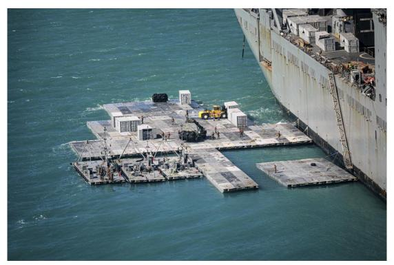
Pictured: US Army mariners construct a "Joint Logistics Over-the-Shore" causeway adjacent to the MV Maj. Bernard F. Fisher off the coast of Bowen, Australia, July 29, 2023. This is the type of floating pier that the US military has been tasked with building on the Gaza shore. (Photo by Sgt. Ashunteia' Smith/U.S. Army via Getty Images)
